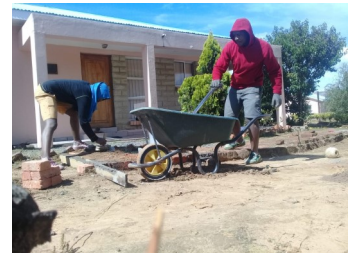
On site staff repairing the centre
